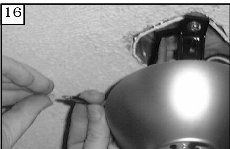
16 Make wire connections to power source using wire nuts provided. Make sure that no filiments are outside of the wirenut. After making the wire connections, the wires should be spread apart with the grounded conductor and the equipment-grounding conductor on one side of the outlet box and ungrounded conductor on the other side of the outlet box.
